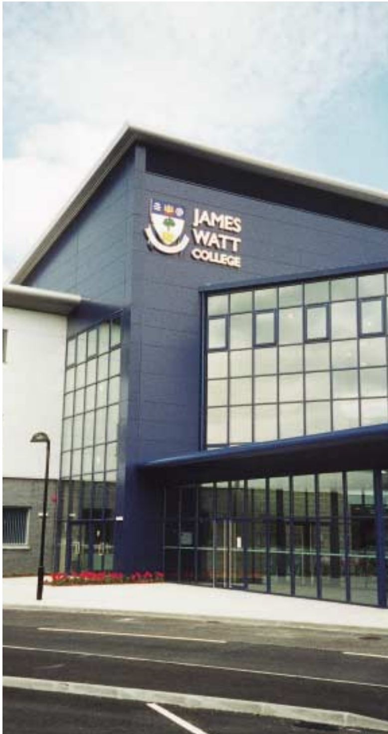
FRONT ELEVATION SHOWING THE ATRIUM OF THE NEW NORTH AYRSHIRE CAMPUS FOR JAMES WATT COLLEGE AT KILWINNING. THE COLLEGE WAS COMPLETED IN JUNE 2000 AND THE FIRST STUDENT ENROLMENT TOOK PLACE IN AUGUST 2000.
